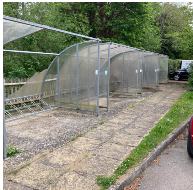
The long-term cycle parking at residential flats provided in the form of shelters with wheel slots. The provision does not allow for a bike frame to be locked to anything, and the proximity of a public footpath behind the site leaves cycles left there vulnerable to theft.
