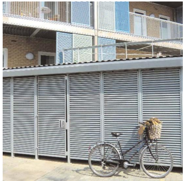
A secure cycle parking compound at a block of flats.
