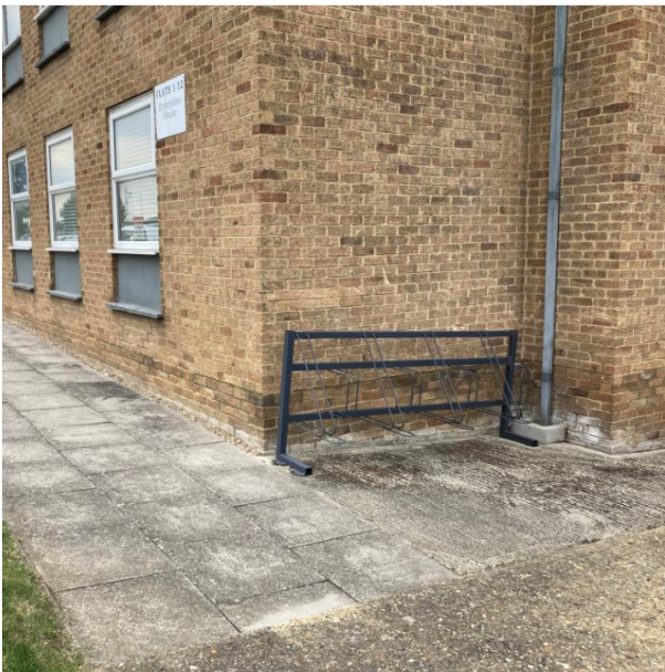
Cycle parking provision at a commercial building that has been converted into residential apartments. The cycle parking is not covered, does not provide a fixed bar for the frame of the bike to be locked to and is not overlooked by any of the properties in the building.
