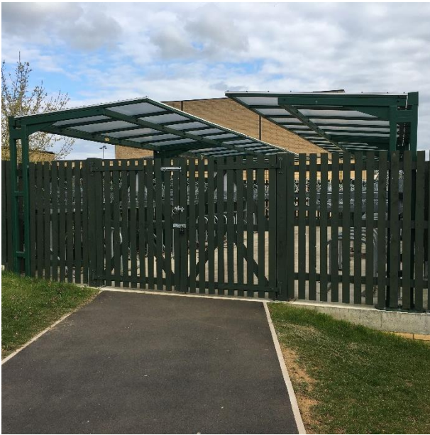
A secure cycle parking area at a secondary school. The area is fenced and covered with a lockable gate, and incorporates a combination of Sheffield stands and two tier cycle racks.
