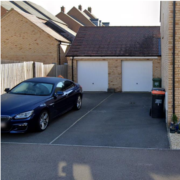
Properties designed with limited frontages and no rear access result in wheelie bins stored in driveways, and vehicles parked on-street.
