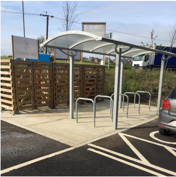
Cycle parking provision squeezed into the corner of a car park. If vehicles are parked in both spaces adjacent to the cycle parking area, access to the cycle parking (and bin storage behind) is restricted.
