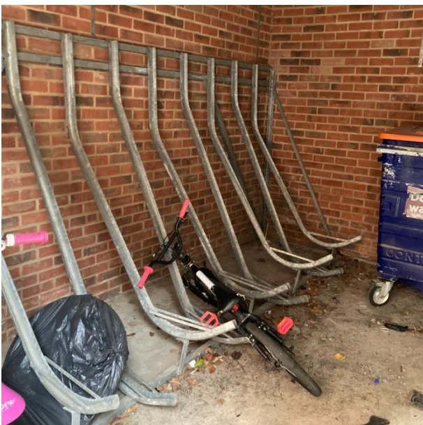
Cycle parking racks for long-term parking at residential flats combined in a brick-built bin store. Bins and cycles should be accommodated in separate locations. Some of the cycle racks are not accessible due to the bins and rubbish has been dumped in between the cycle racks.
