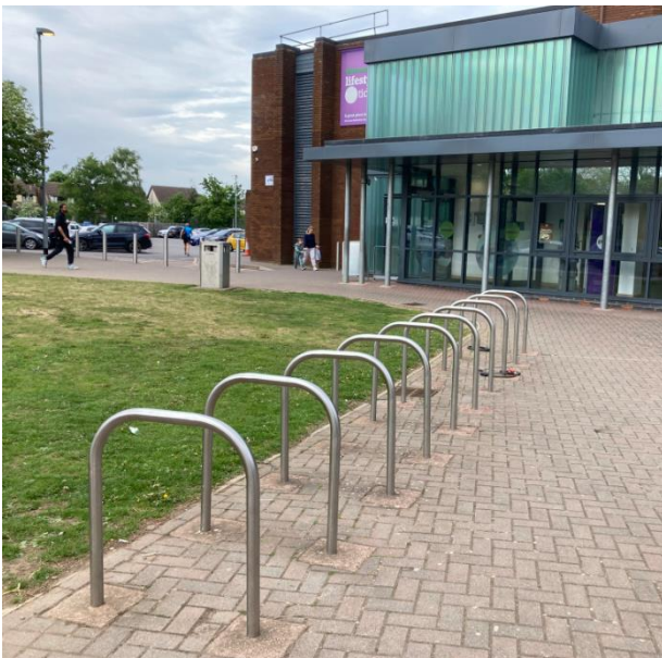
Cycle parking outside a leisure centre where Sheffield stands have been installed too close to the edge of the block paved area, meaning that bikes locked here would be partly on the grass.
