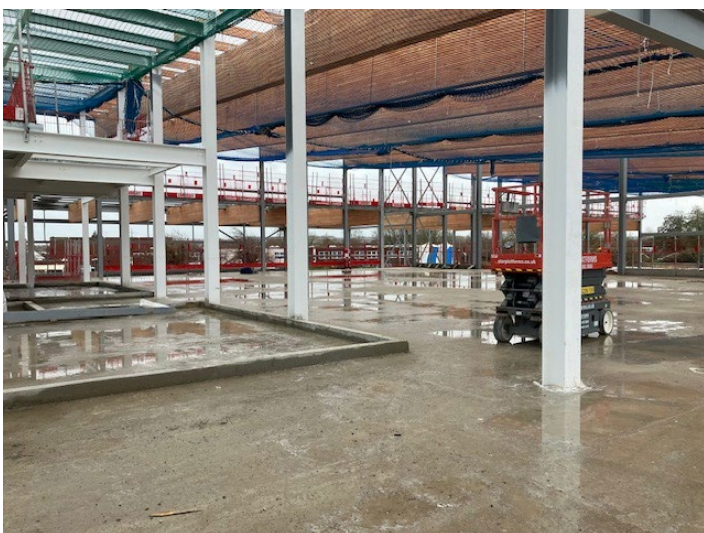
First Floor Slab
